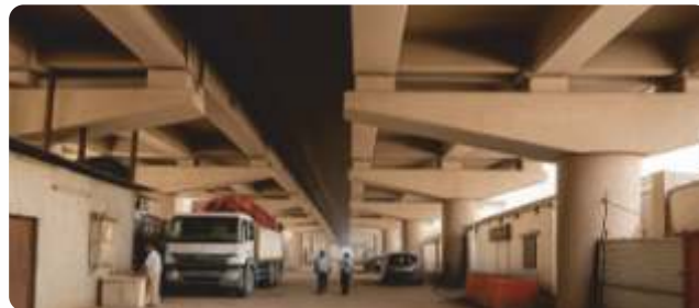
Repair & Retrofitting of Bridges in Mumbai MH
