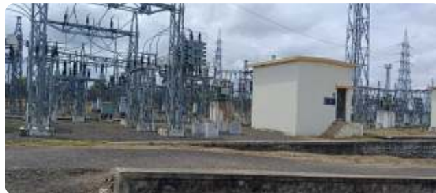
Substation Augmentation at Sakoli, Bhandara, MH | 132kV
