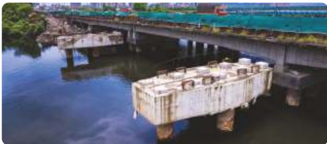
Taloja Creek Bridge, Panvel MH | 130 M
