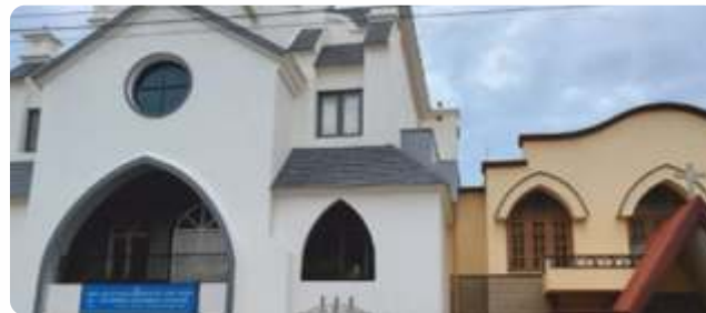
Retrofitting of Bettel Thoma Church Bengaluru KA
